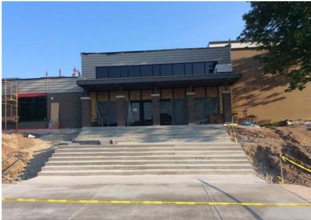
Main Entrance of School
