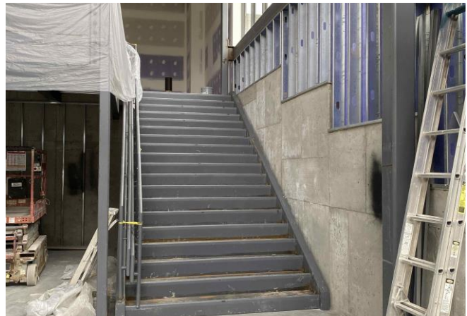
Fitness Center Entrance Stairs and Lobby
