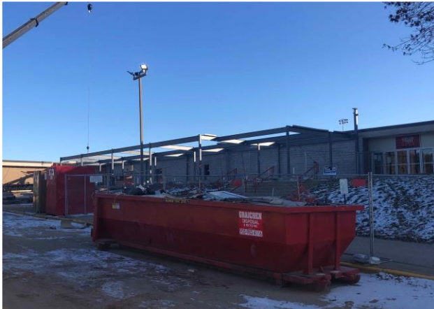
Structural steel being erected
