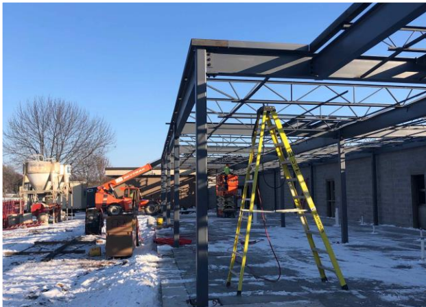
Steel joist install
