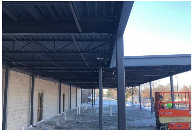
Decking installed over steel joist
