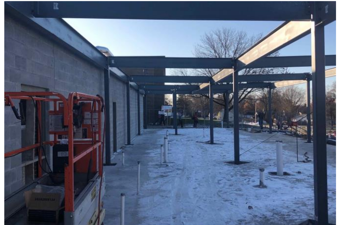
Structural steel ready for joist install
