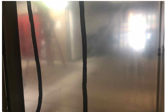
Plastic partitions close of construction areas
