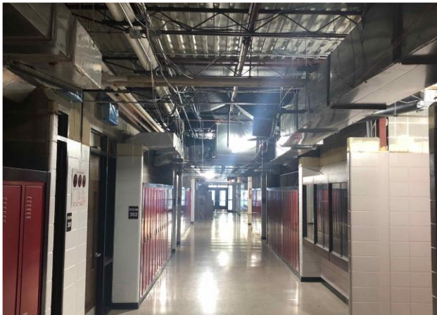
Corridor renovation work is underway 2 nd shift
