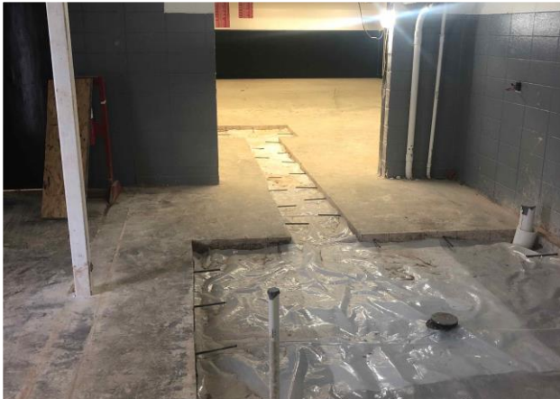
Lower level underground work complete
