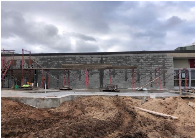
Finished Masonry Wall Admin Addition.
