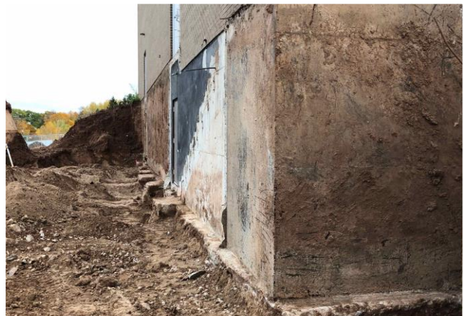
Excavation completed in Fitness Center.
