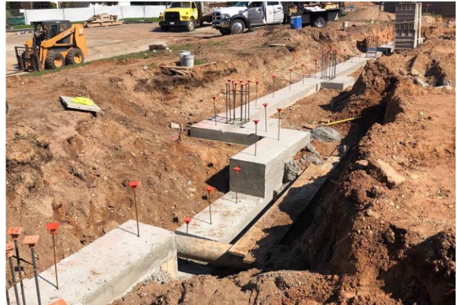
Footings and rebar installed Admin Addition
