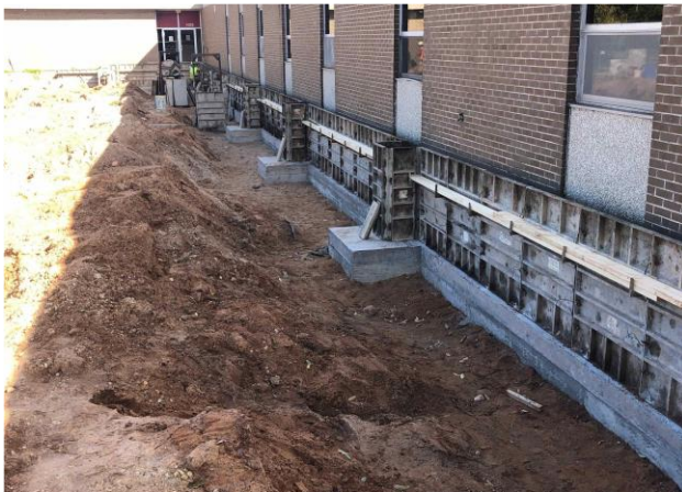
Foundation wall forms installed Admin Addition
