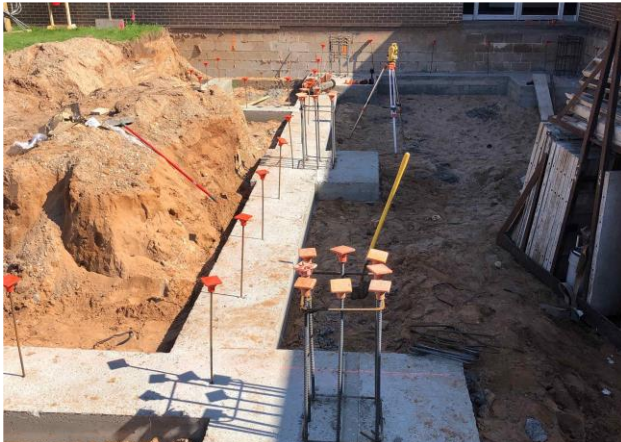
Footings and rebar installed Admin Addition
