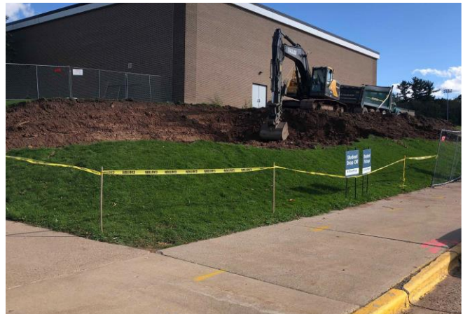
Sanitary Sewer Install
