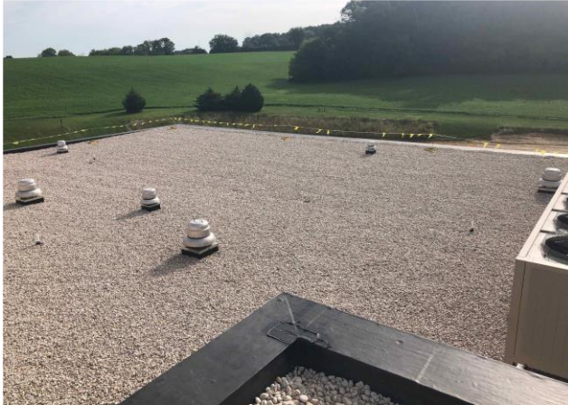
New Roof Complete at MES
