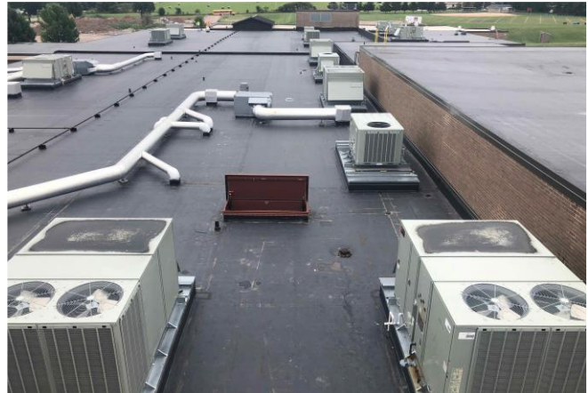
New Roof Complete at High School
