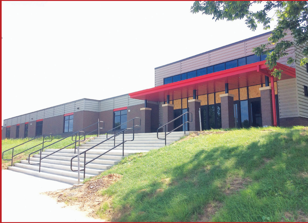
NEW FRONT ENTRANCE WITH ADMINISTRATION SUITES
